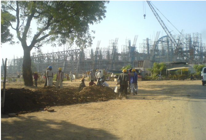
Software Block, L&T Construction Site at Bangalore
