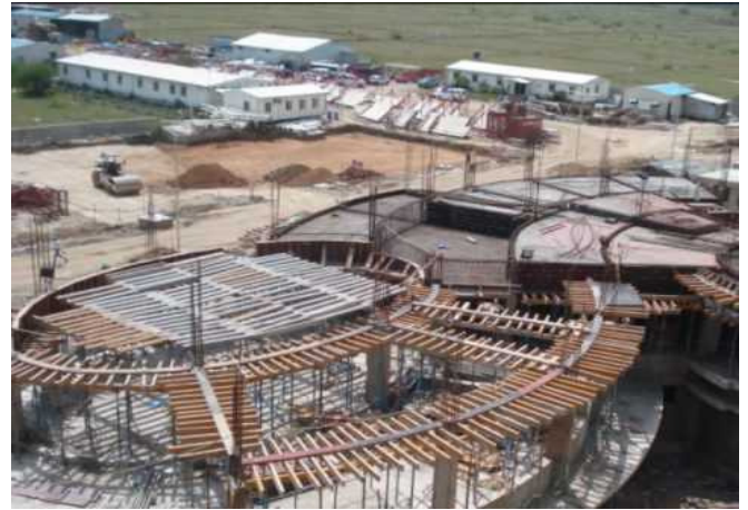
Shuttering Details of Software Development Block at L&T Site, Bangalore
