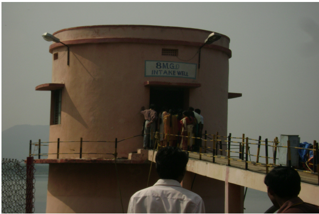
Water Intake Structure of Dr. K. L. Rao Water Works
