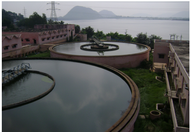
Clarifier of Dr. K. L. Rao Water Works
