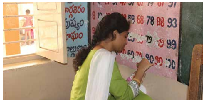
Water curing a brick of wall surface by civil students
