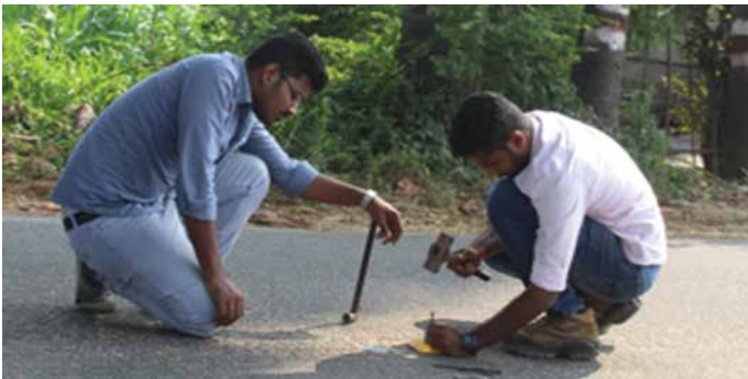
Placing radium-reflector (radium sticker) to make night vision clear for all drivers to reduce night accidents.
