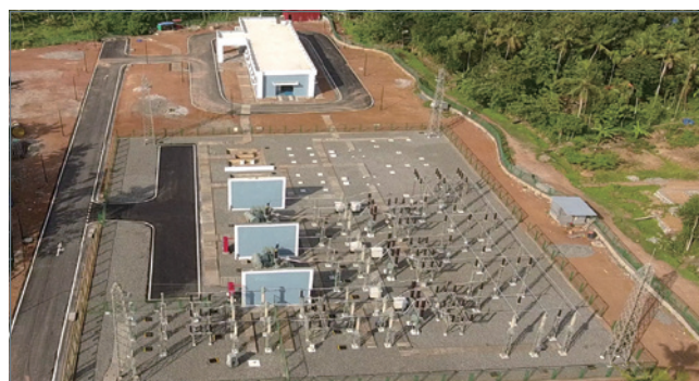
Figure 9-16. Techno Park – Digital Substation
