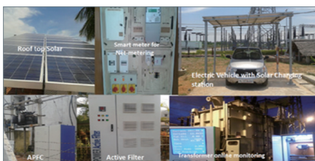
Figure 9-14. Installation of PQM, RE integration, Electrical vehicle at Puducherry
