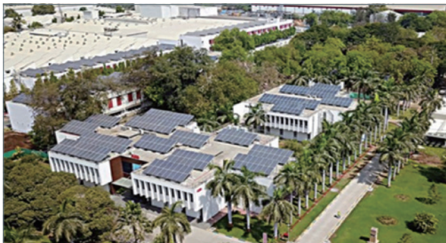
Figure 9-17. Rooftop solar park
