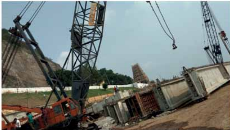
ERECTION OF PRE-CAST GUDDERS
