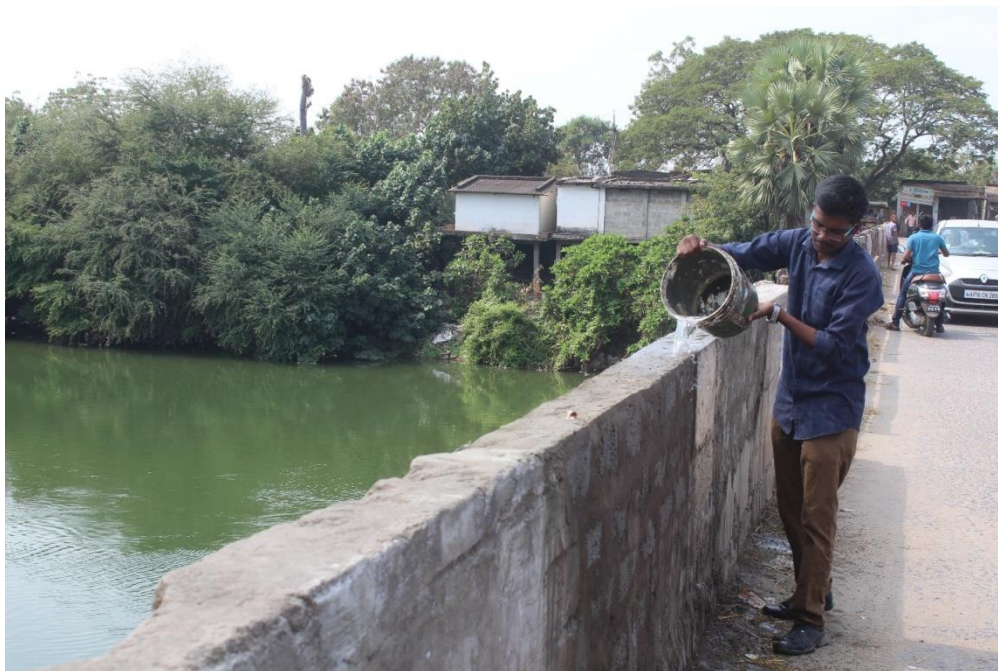
Water curing a brick of wall surface by civil students
