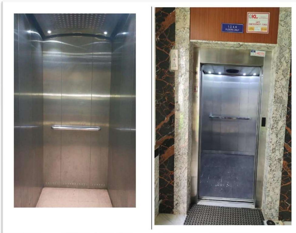
CENTRAL LIBRARY BLOCK LIFT AND RAILING FACILITY
