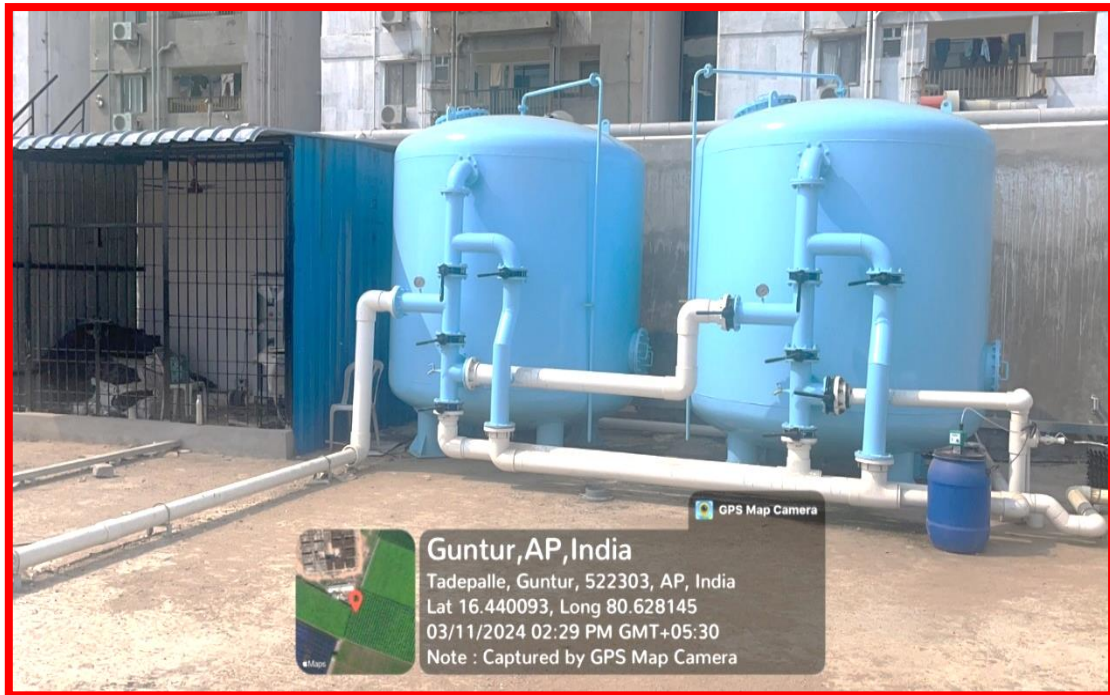
STP-5, Near Tulip Residency, ARBiT Technology, 1200 KLD capacity
