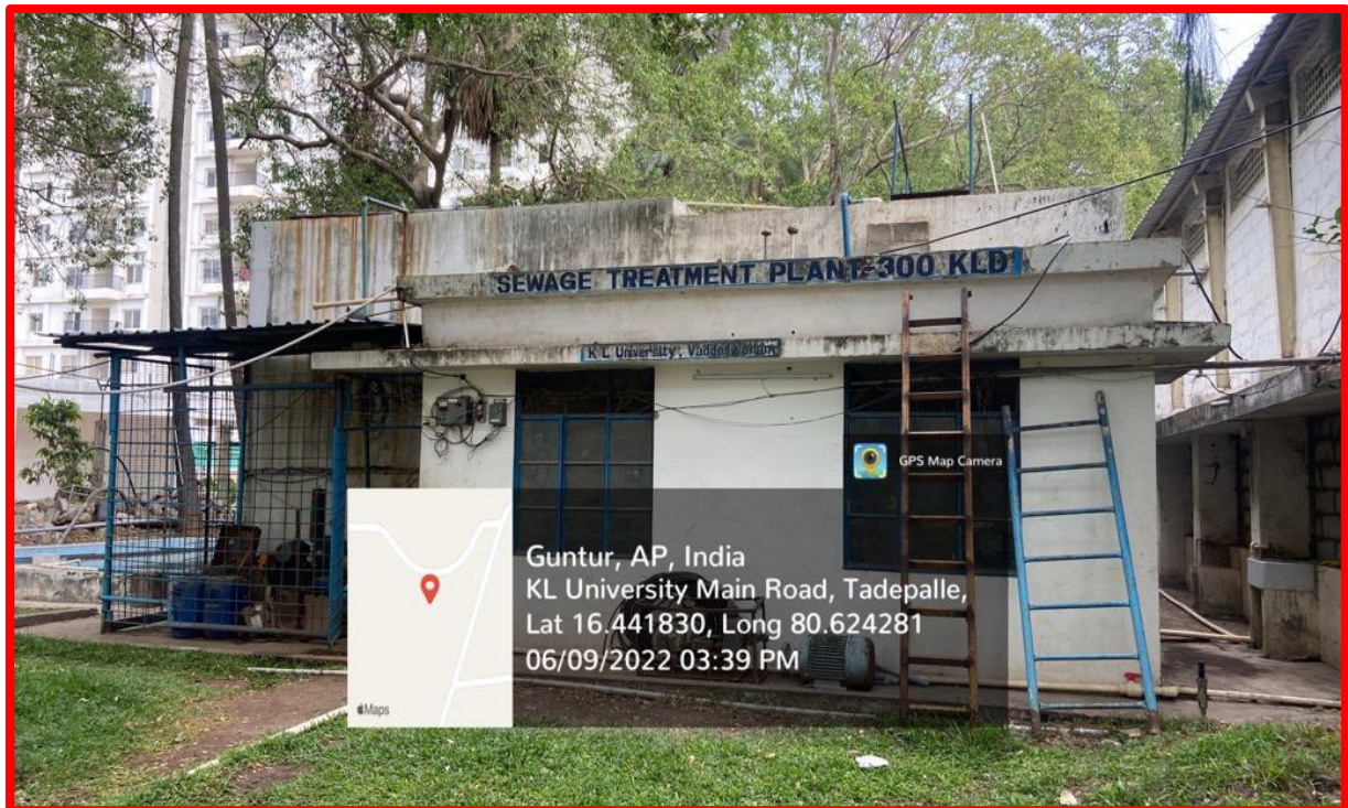
STP-1, Near Main Canteen, MBBR Technology, 300 KLD capacity
