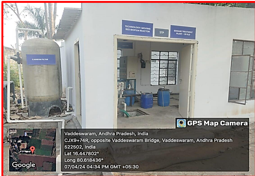
STP-3, Near Nilagiri Girls Hostel, MBBR technology, 30 KLD capacity
