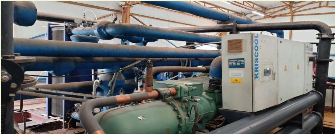
Figure 2: Centralised water-cooled chiller plant
