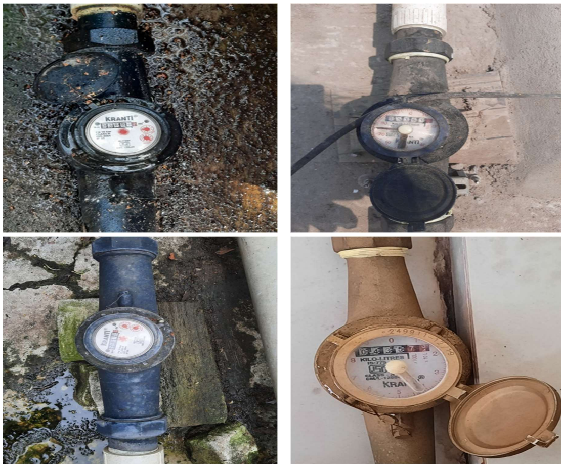
Figure 15: Water meters for recording water use- treated effluent use in STP 1, 3 and 2 and groundwater in one of the overhead water tanks of the block
