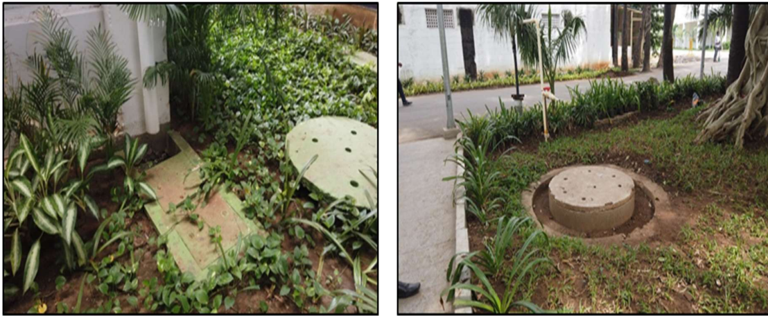
Figure 12: Rainwater recharge pit with desilting chamber
