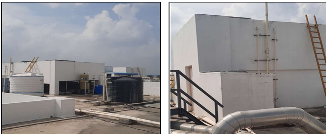
Figure 10: Overhead domestic and fire water tank located on the terrace of one the blocks
