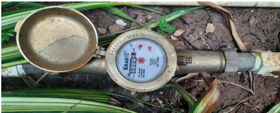
Figure 7: Bore located near the FED block with water meter installed for taking the readings for groundwater extraction
