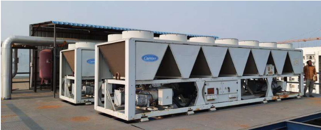
Figure 3: Centralised air-cooled chiller plant
