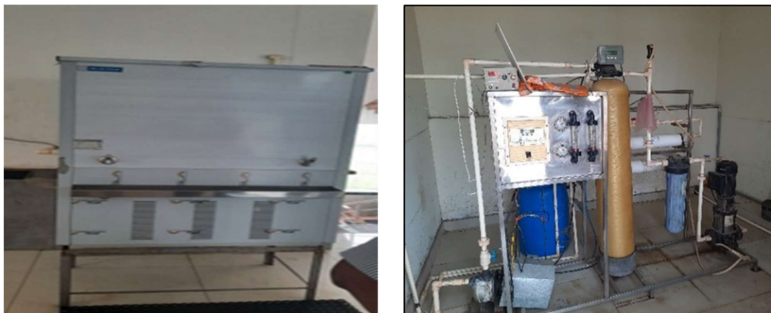
Figure 8: RO plant installed on the terrace of one of the blocks and a water cooler on the ground floor for drinking water
