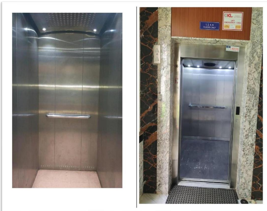
CENTRAL LIBRARY BLOCK LIFT AND RAILING FACILITY
